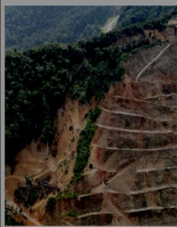
Figure 3.14a: Slope cutting along highway route (extracted from the Landslide Study at CH23+800 Simpang Pulai – Lojing Highway Malaysia Report submitted by Andres Malone Ltd (May 2007)
