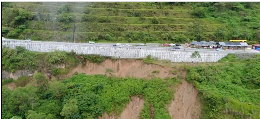
Figure 3.16: Mitigation measures – piled embankment undertaken to reduce the impact of landslide
