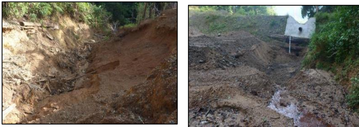
Figure 3.19: Dumping of the soils along the slope and uncomplete discharge point into the slope towards the water catchment area in 2013
