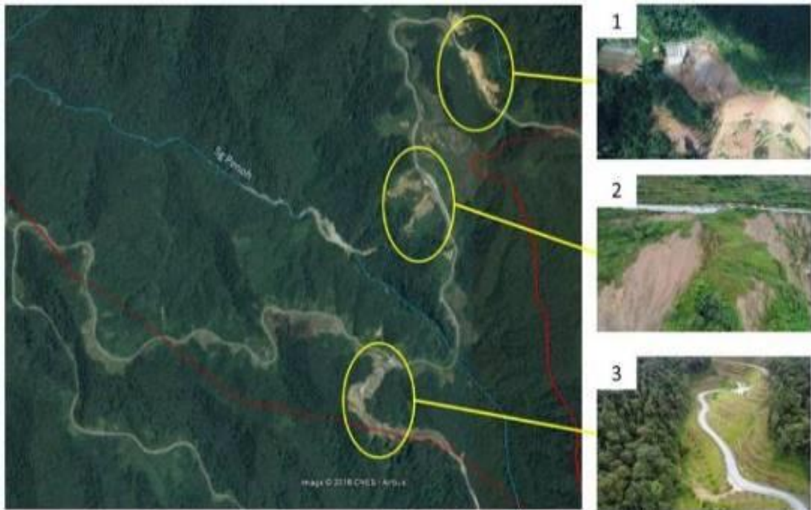
Figure 2.3: Satellite image and drone photo of the landslide and the erosion ending up into the Penoh River feeding into the Kinta River and finally into Sultan Azlan Shah Dam
