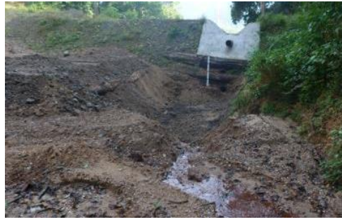
Figure 3.20 Dumping of the soils along the slope and incomplete discharge point into the slope towards the water catchment area in 2013
