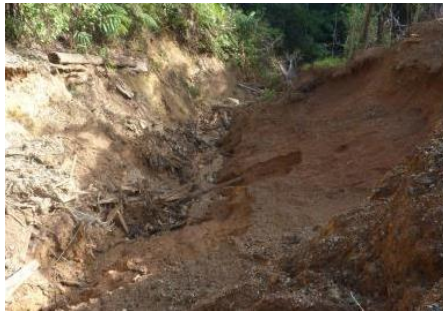
Figure 3.20 Dumping of the soils along the slope and incomplete discharge point into the slope towards the water catchment area in 2013
