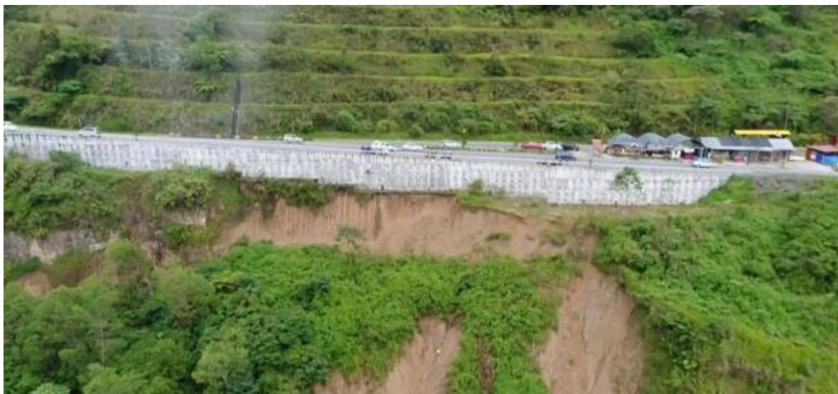
Figure 3.15 Mitigation measures – piled embankment undertaken to reduce the impact of landslide
