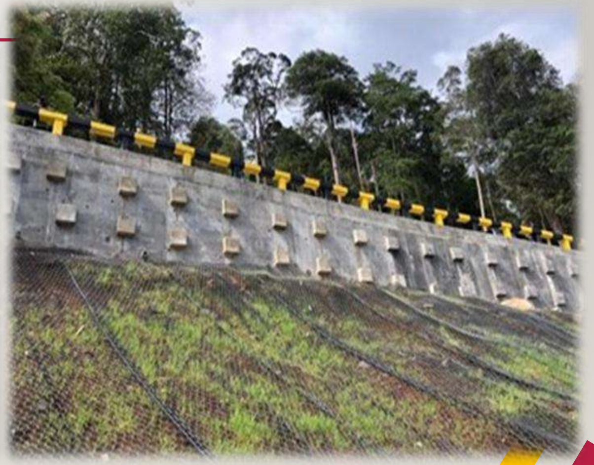
Tie Back Wall
